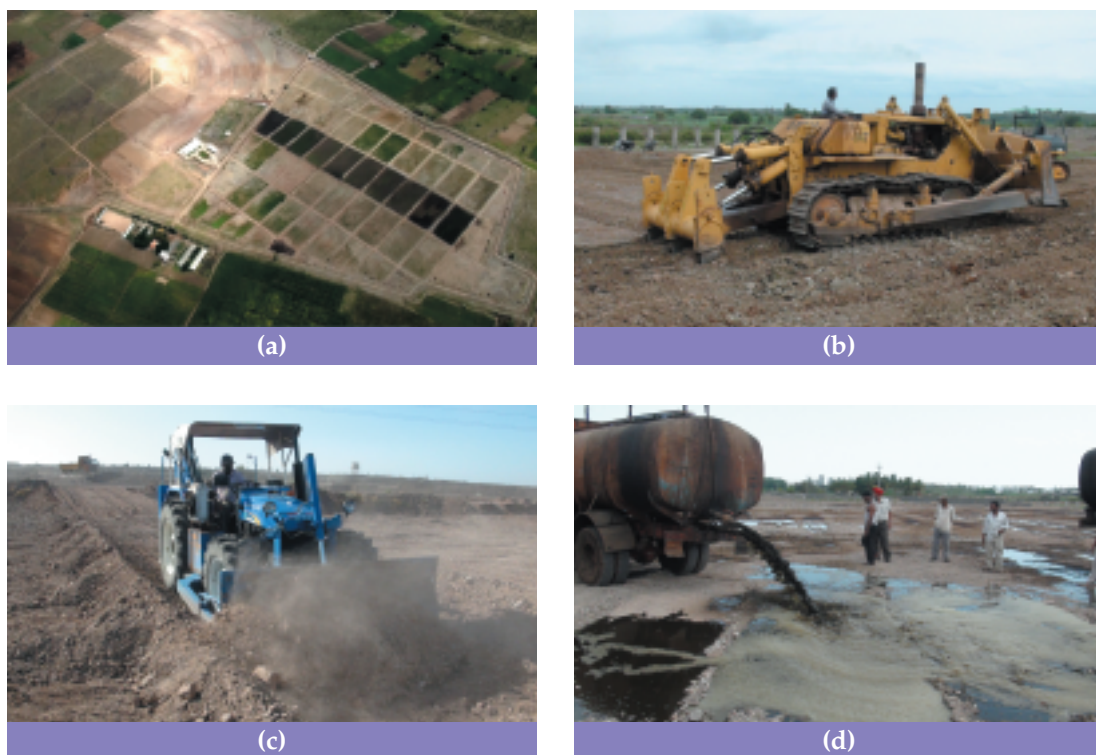
Fig. 2.5. Aerial view of the Research Farm (a), A 350 hp dozer-ripper preparing terraces by ripping and levelling (b), Preparation of farm paths using 75 hp tractor mounted dozer attachment (c), Spent wash being applied for developing research plots (d)
