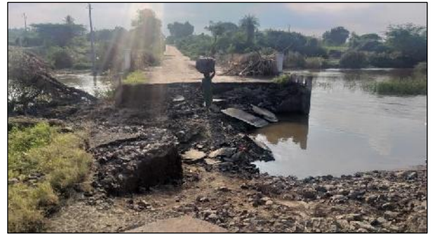
Damaged/broken road bridge over big stream
