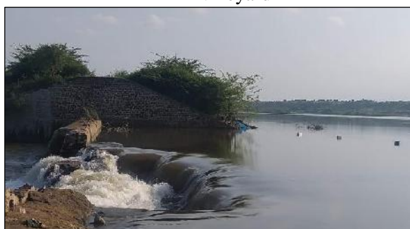
Collapsed embankment of Lake
