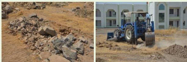
Soil showing hard stones on opening of pits
