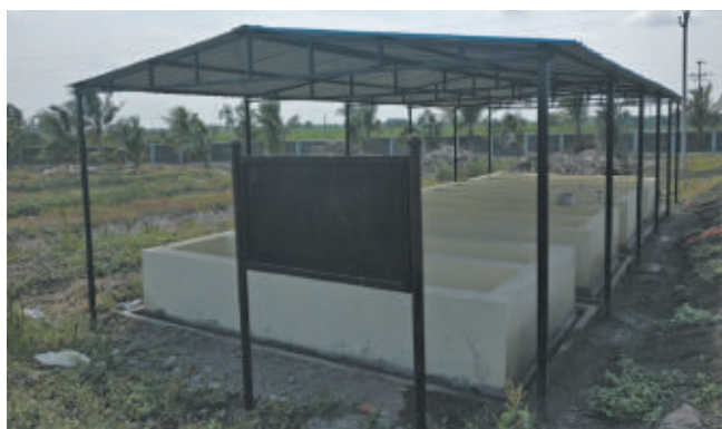
Vermicomposting unit under construction
