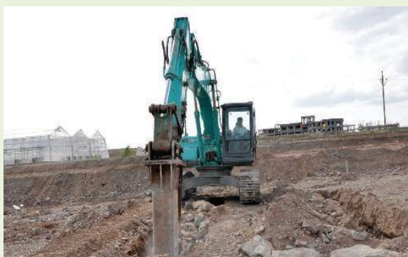
Ripping/chaining of rocky surface
