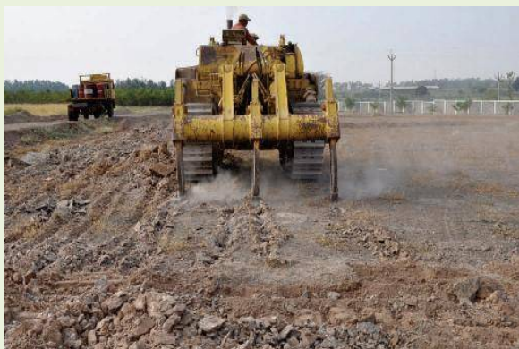
Ripping/chaining of rocky surface
