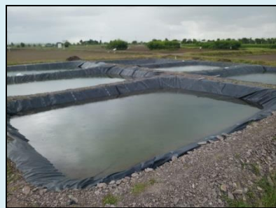
Lining of ponds with HDPE sheets
