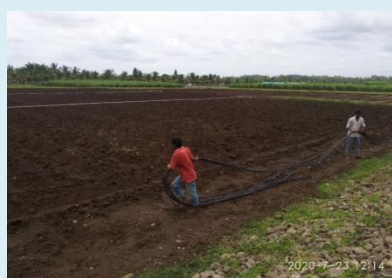
Installation of sub surface drip irrigation
