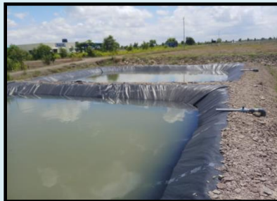
Lining of ponds with HDPE sheets
