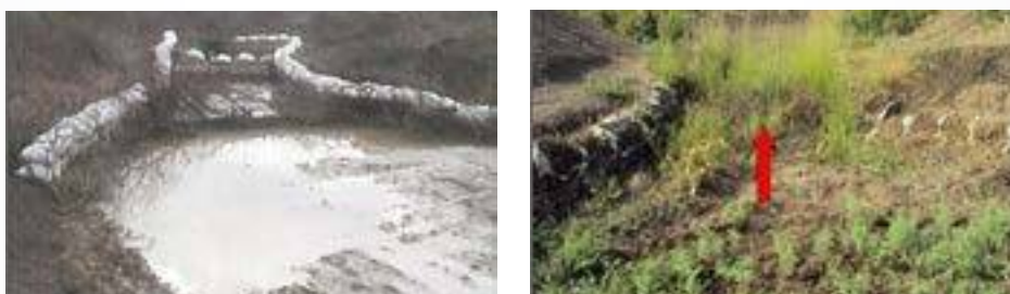
Figure 6.19 : Technology (Brushwood inlet spillway) developed under NAE programme for the protection of inlet of farm pond
