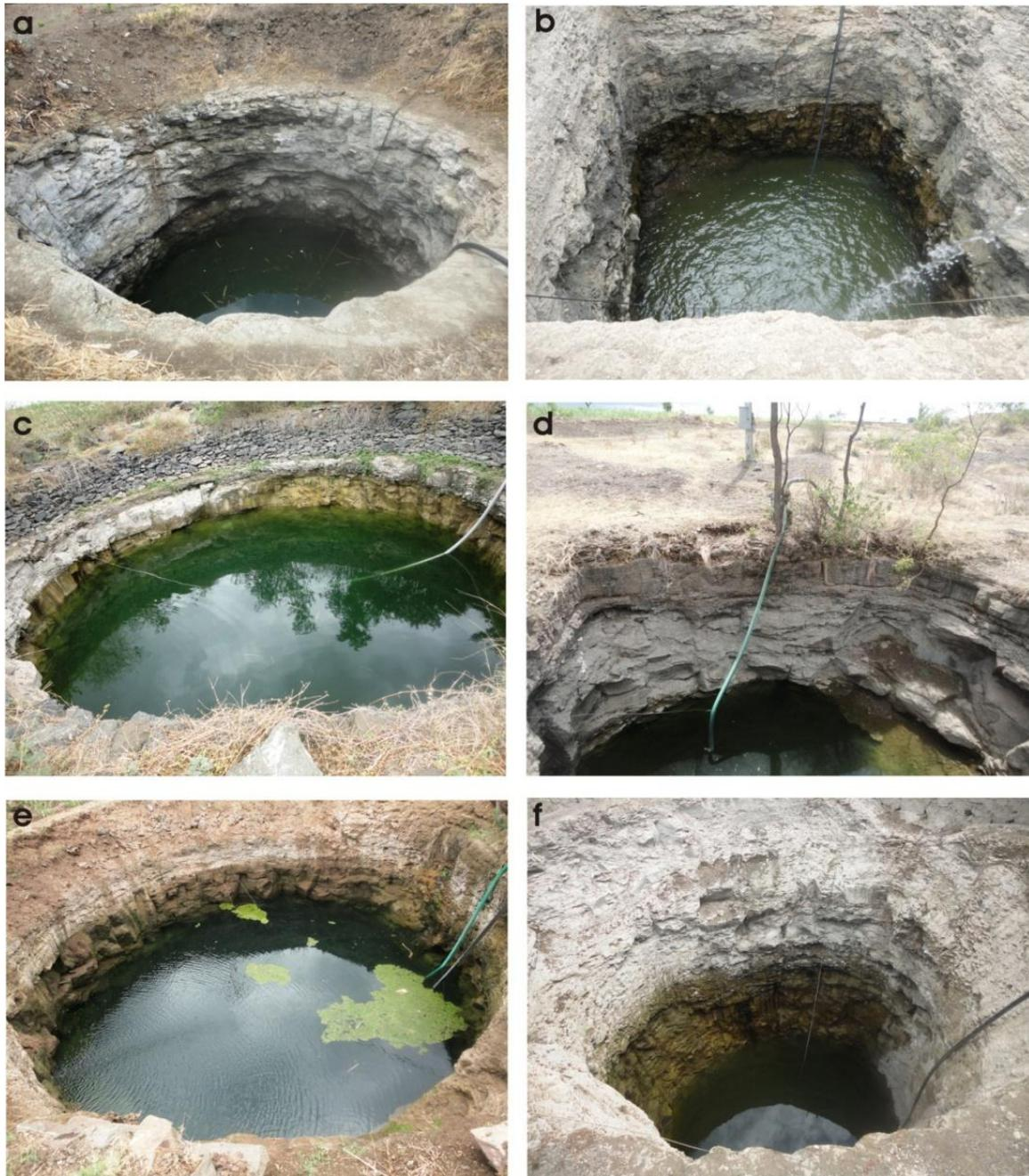
Fig. 2.7 Field photographs of water abstraction structures (dug wells) from the study area
