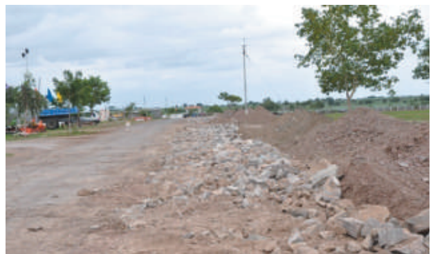
Application of murum and completed East-West road
