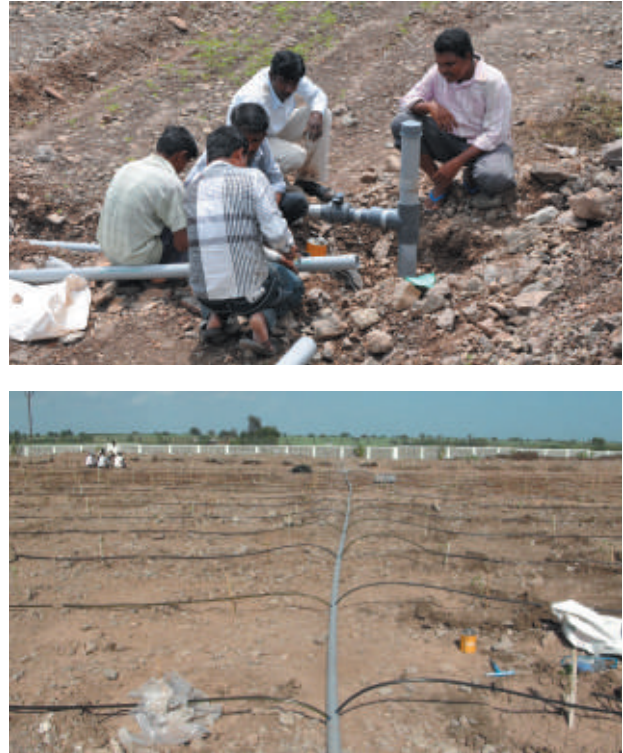
Fig. 23. Installation of drip irrigation system in north-east farm
