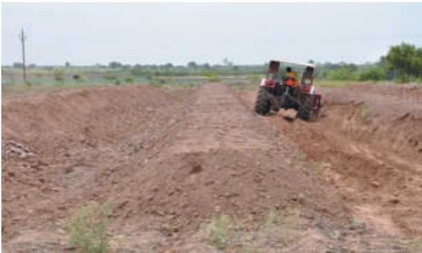
Levelling trenches between raised broad beds
