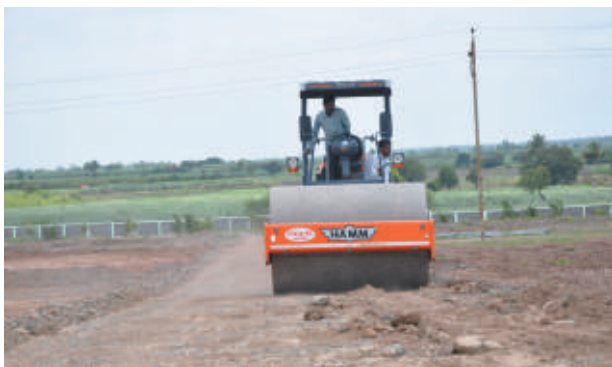
Pressing of murrum layer with road roller
