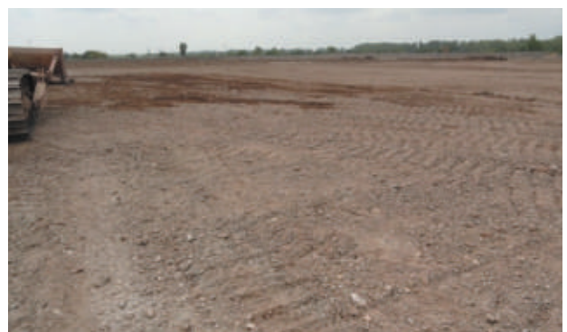
Levelled, ripped and chained field
