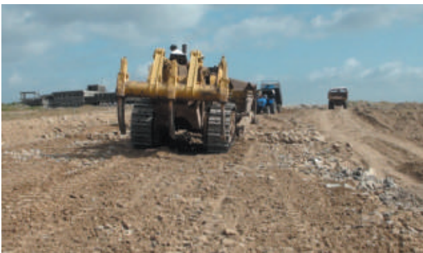
Application of murrum and completion of road work
