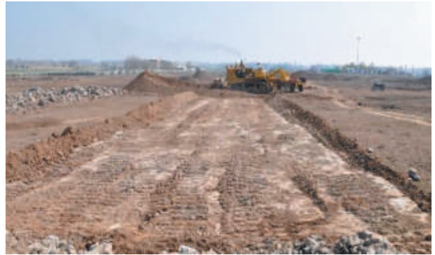
Scraping of murrum and road demarcation
