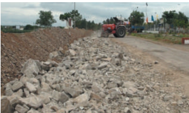
Application of murum and completed East-West road
