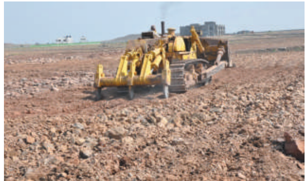
Ripping after blasting
