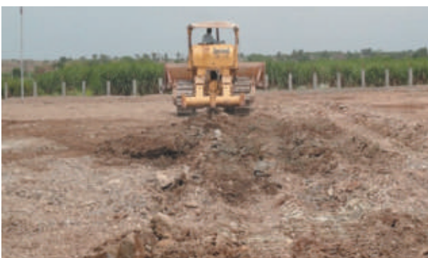
Second ripping and chaining operation
