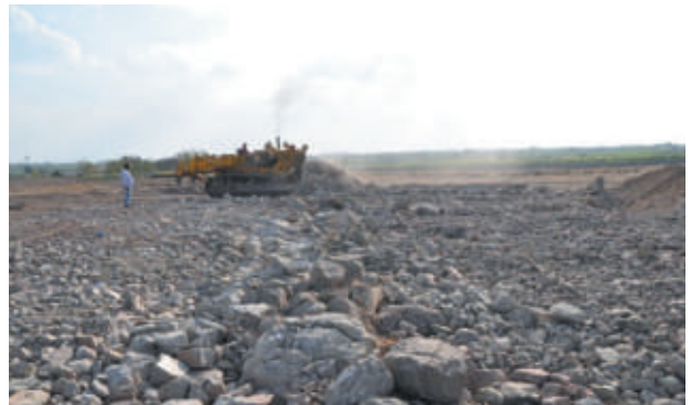
Chaining and pressing of boulder
