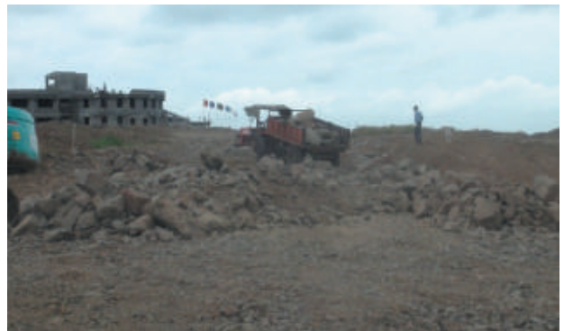
Dumping and filling with boulders
