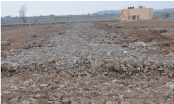
Road after first chaining by dozer
