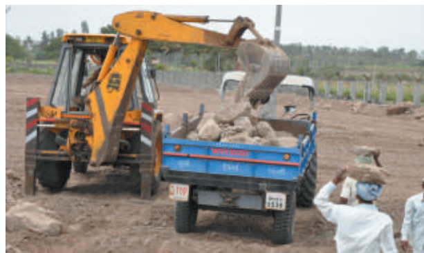
Collection of stones for road filling
