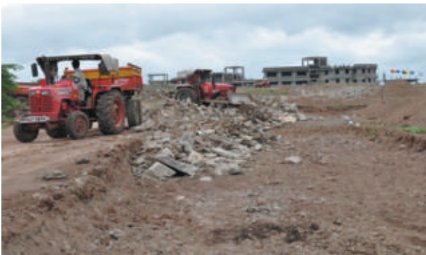
Dumping and filling with boulders
