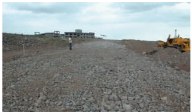
Dumping and filling with boulders
