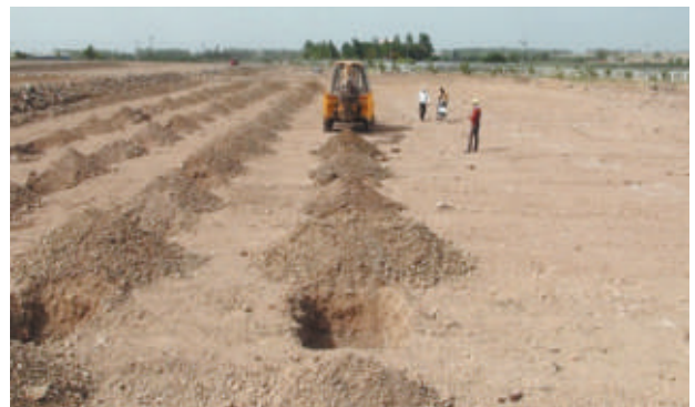
Making pits using JCB
