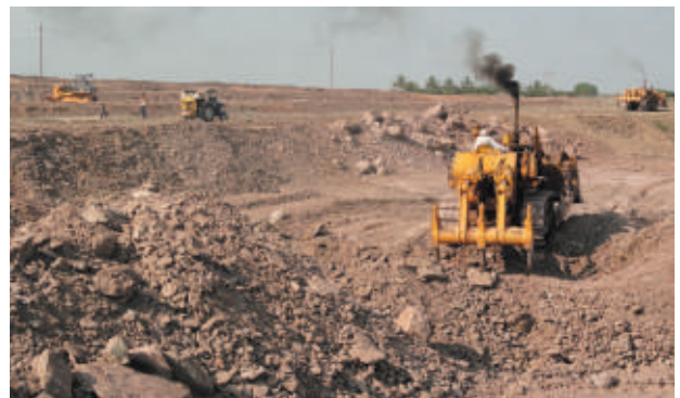
Ripping/chaining of rocky surface
