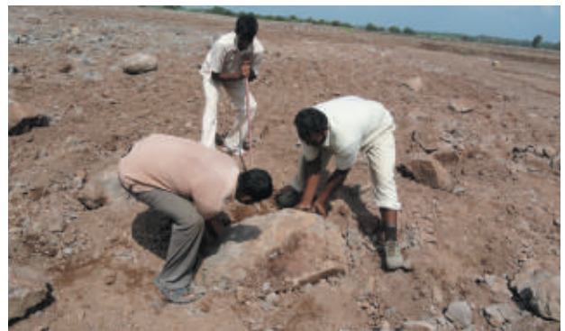
Removal and collection of the heavy boulder for road filling
