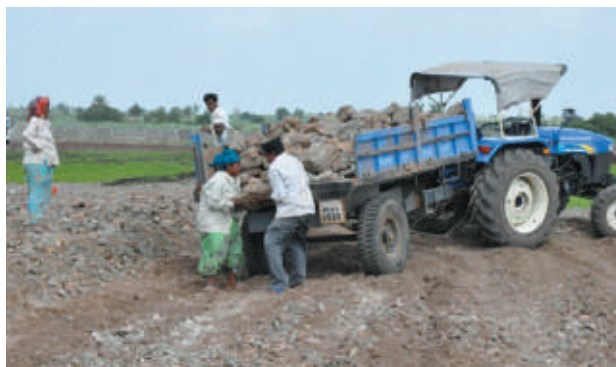
Removal of stones before levelling work
