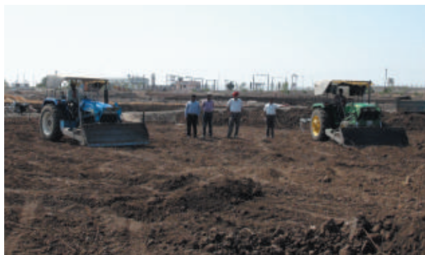
Fig. 13 Import, filling and levelling of black soil for preparing field for field experimentation
