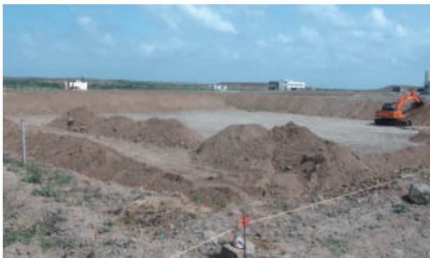
Fig. 29. Construction of water balancing tank in northern side
