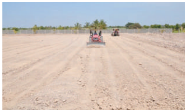
Complete rough levelled murum plot
