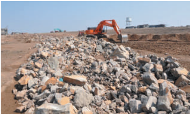
Dumping and filling with boulder
