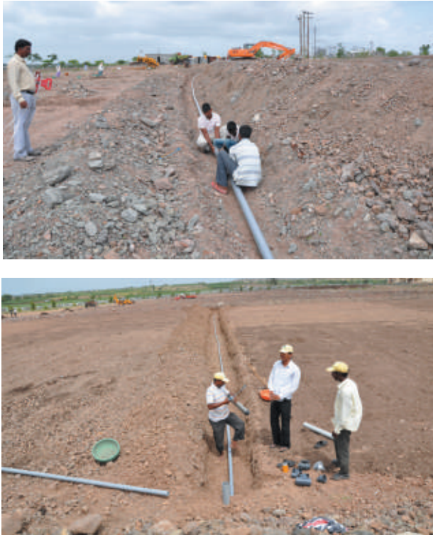
Fig. 23. Installation of drip irrigation system in north-east farm
