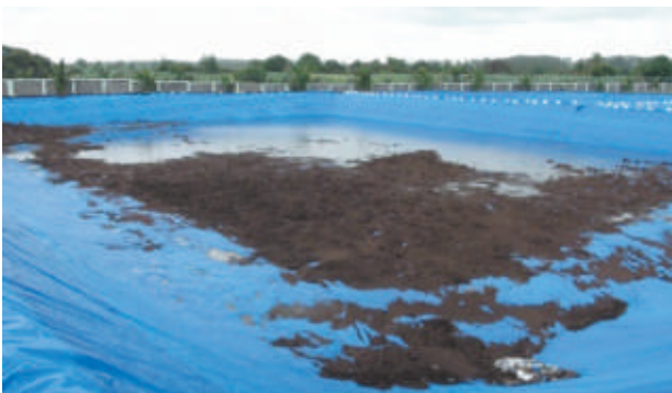
HDPE Lining to prevent seepage
