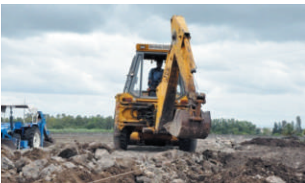
Setting of boulders in line for road
