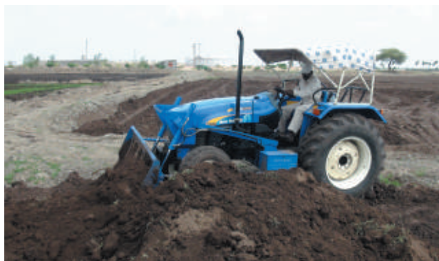
Fig. 13 Import, filling and levelling of black soil for preparing field for field experimentation
