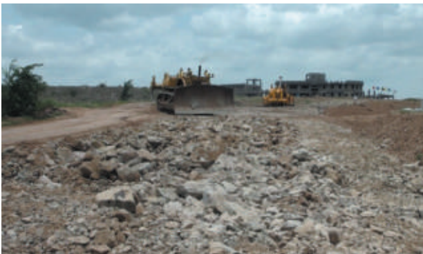
Dumping and filling with boulders
