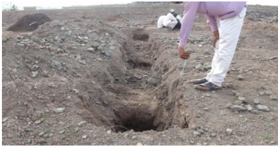
Depth of normal pit after blasting
