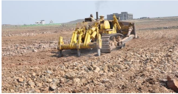
Ripping and chaining with heavy machineries
