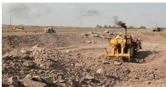
Step 1: Ripping/chaining of rocky surface
