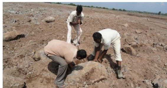
Step 3: Removal and collection of the heavy boulder for road filling
