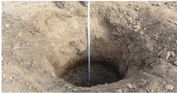
Depth of auger pit after blasting
