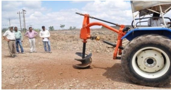
Making pits with post hole digger
