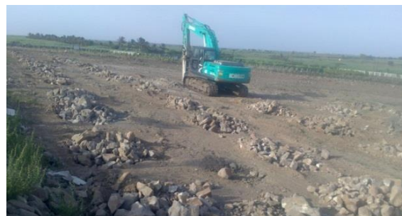
Making pits with Pokhlain/JCB
